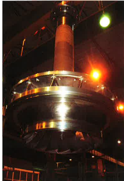
Figure 2 – Guthega Stator Lift
